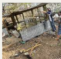
Roofing and Siding
